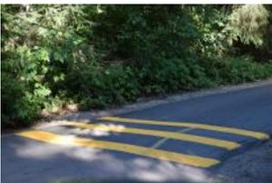
**Description of Photo 3 : Example of speed bump on roads around campsites - bright contrast and thick lines painted for increased visibility**
