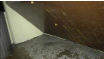
**Description of Photo 4 :** Plate under sink insulates the pipes but might interfere with getting close enough for some wheelchairs
